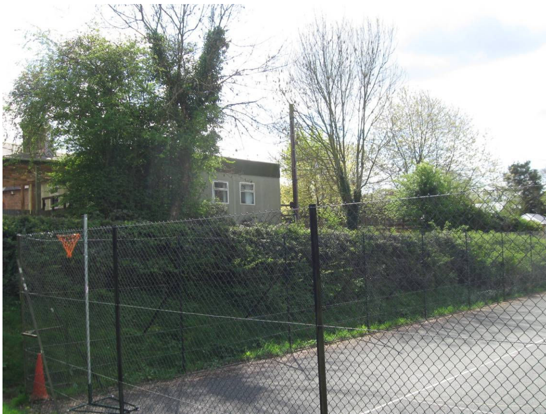
Photograph of existing mobile classroom from playing fields looking south
